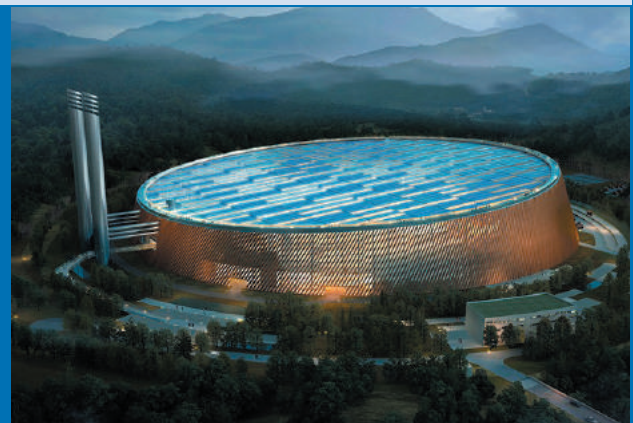
Shenzhen East WtE plant with solar panel rooftop.
