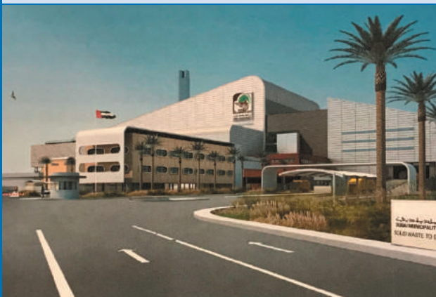
Dubai WtE plant.
